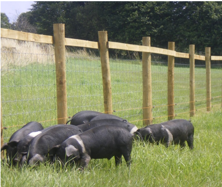
Fig 1: Our fence – you can clearly see all of the aspects of the fence, posts, mesh, top rail and electric wire.
